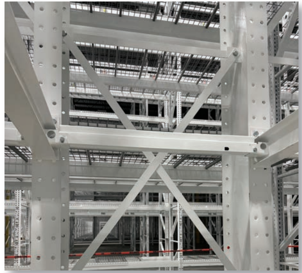
Bracing - Pre-punched holes for bolting to bracing clips on the columns.
