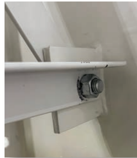
Bracing - Pre-punched holes for bolting to bracing clips on the columns.
